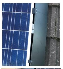
b. Some bigger end clamps (Variosole clamps that we have seen) are too big for the skirt but can easily be dealt with by cutting out a small notch out of the skirt
